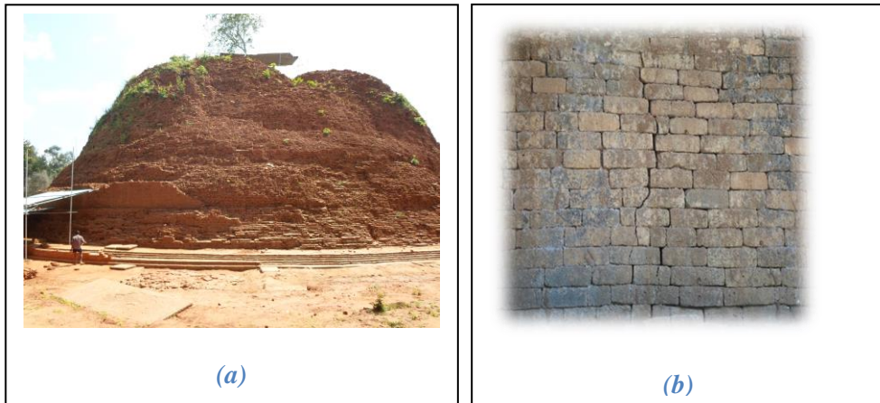
Figure 1. Two views of the stupa: (a) after the removal of vegetation cover (b) a crack formed in the dome of the stupa
